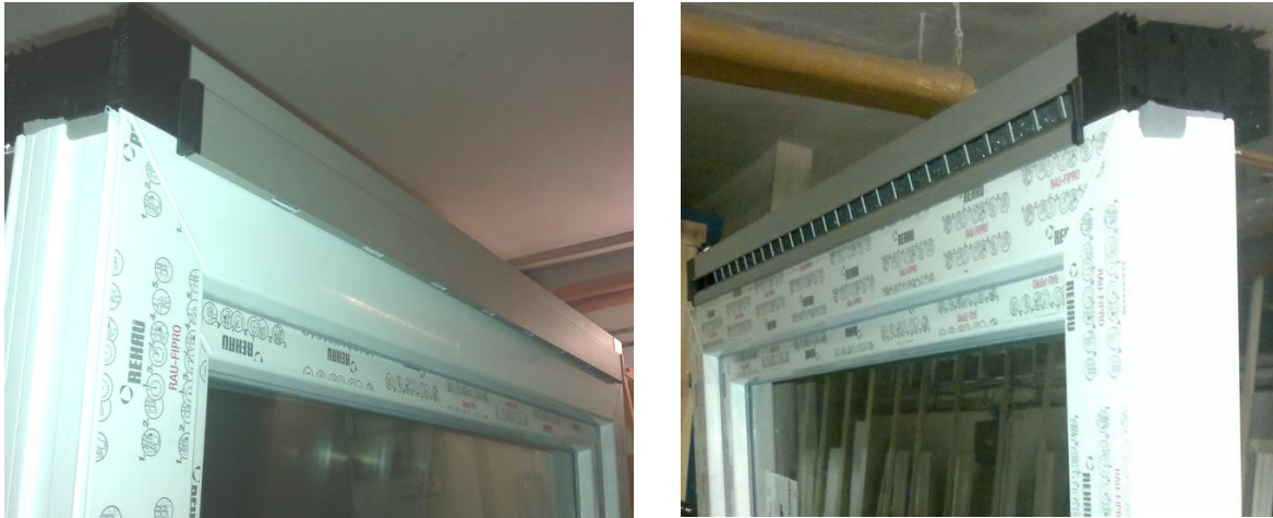
Figure 4. Exterior view of the inlet vent flap installed on the window frame where you can see the inlets of the vent flap type Renson Invisivent AKD Max (left) and Renson Invisivent AK Basic (right).
