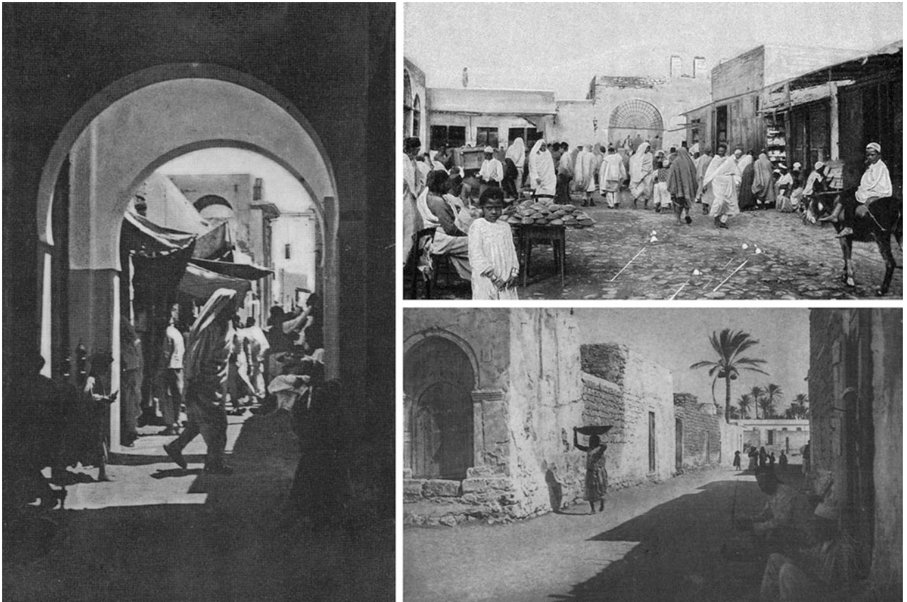
Fig. 6.76 Market scenes (photograph on the left Laronde 1997, photograph on top right Mathuisieulx 1912) and a street in Banghazi during the Italian occupation (Laronde 1997)
