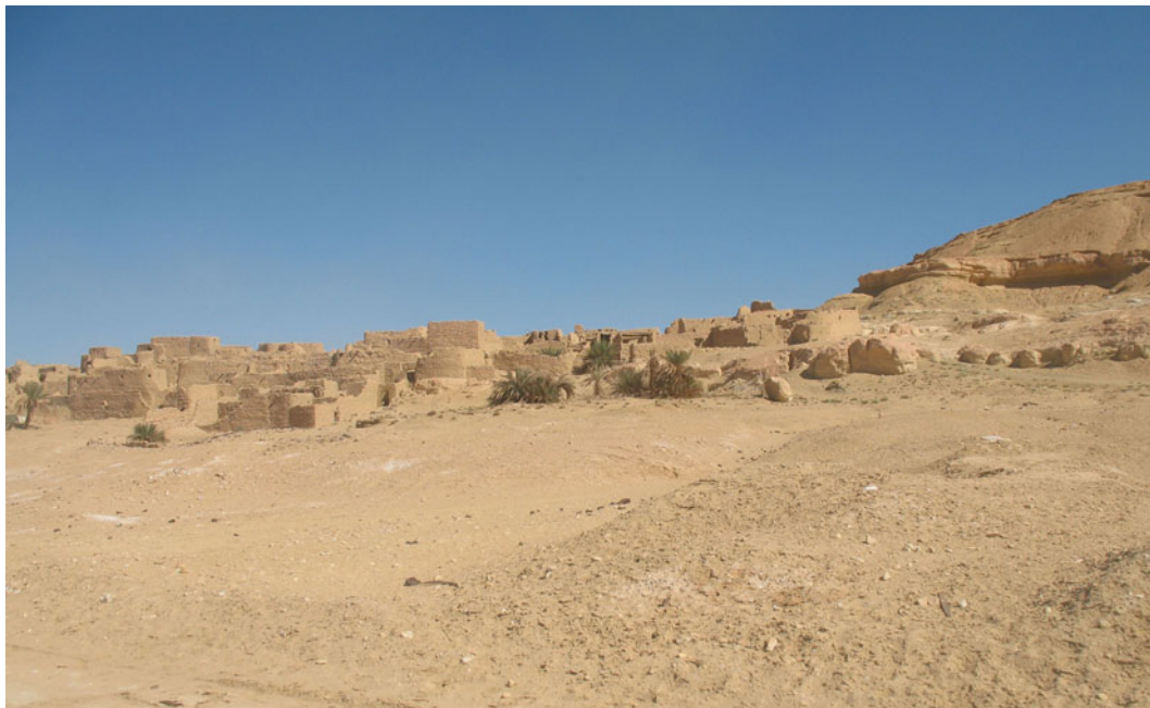
Fig. 6.50 Old town of al Fugaha
