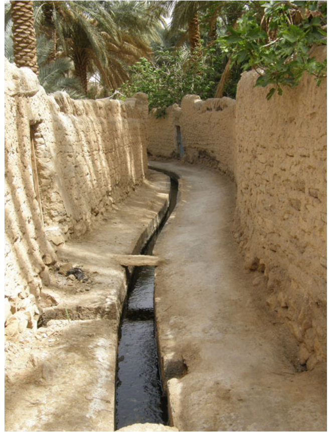
Fig. 6.34 From Ain al Faras, the water runs via water lines to the houses and gardens
