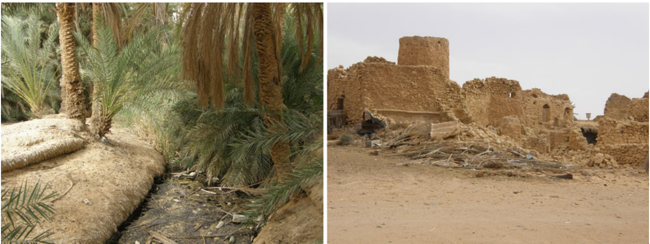
Fig. 5.10 Dams and canals were constructed in order to allow for an all-season irrigation of the gardens of Sinawin. On the right: remains of the old town of Sinawin a formerly important crossroads of the caravan trade
