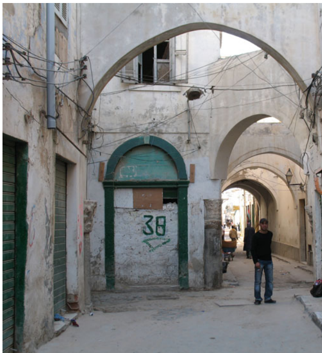
Fig. 6.3 Four-column street, Arbaa Arsat 1 in the Medina of Tripoli
