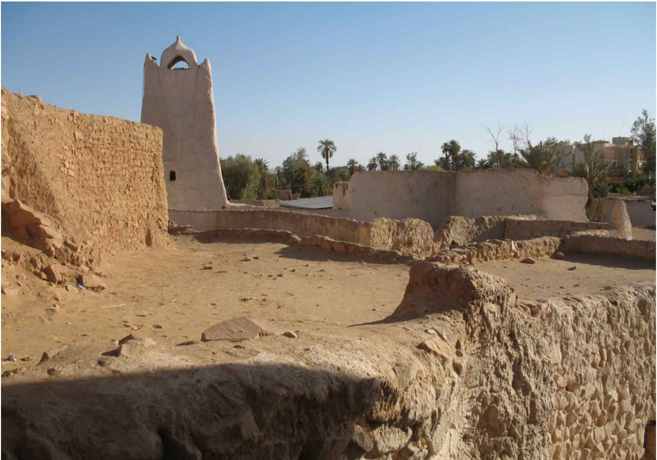
Fig. 6.65 Old town of Ghat is built at the foot of Cocaman Mountain, which situated to the north, holding the fortress, which was initiated by the Ottomans and reconstructed later by the Italians
