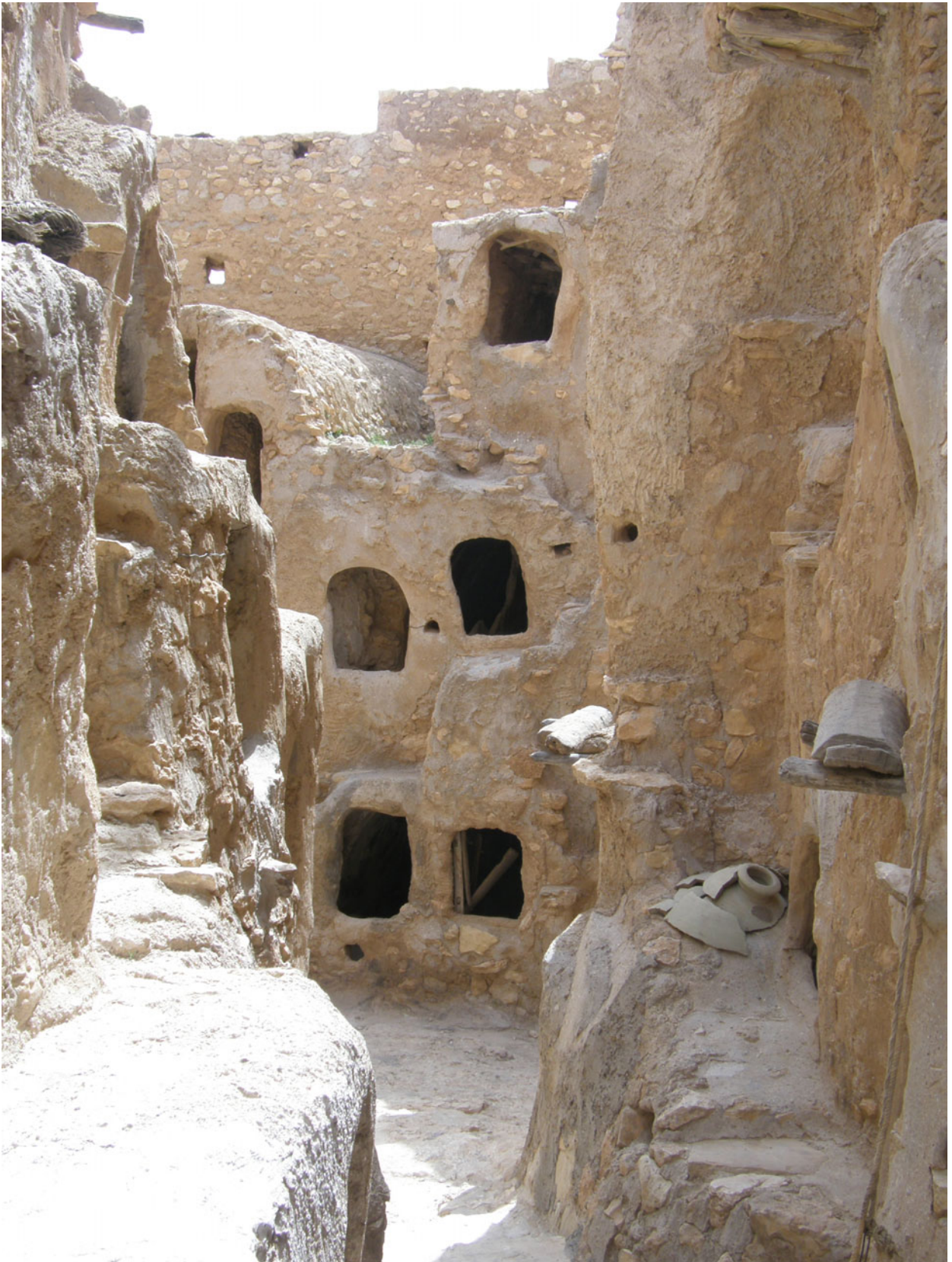
Fig. 6.29 Nalut once linked the routes from Tripoli, Ghadamis and Tunisian cities. The qsar Nalut was a communal building, which housed more than 400 rooms, where local families could store their grain, olive oil and dried fruits. Next to the qsar, there are still houses in local style and several mosques
