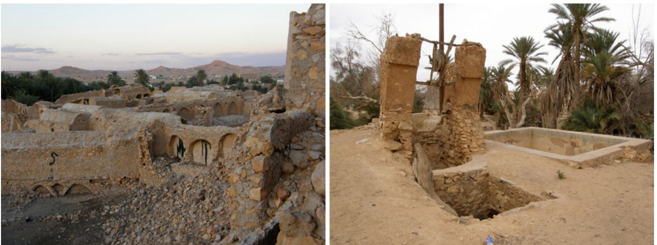
Fig. 6.43 Mizdah has some old houses that mark the old town (photograph on left). A well situated right on the edge of the old city
