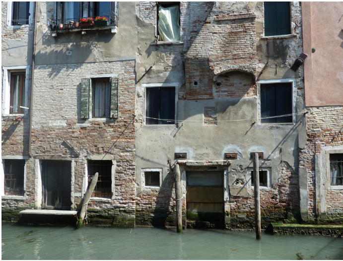
Figure 10.3: The continual morphological computing processes of the elements and marine organisms have weathered these Venetian buildings. Natural forces operate on the fabric of Venetian buildings in complex ways, such as brickwork being digested, generating a coating of white salt or efflorescence. Photograph, Rachel Armstrong, August 2010.
