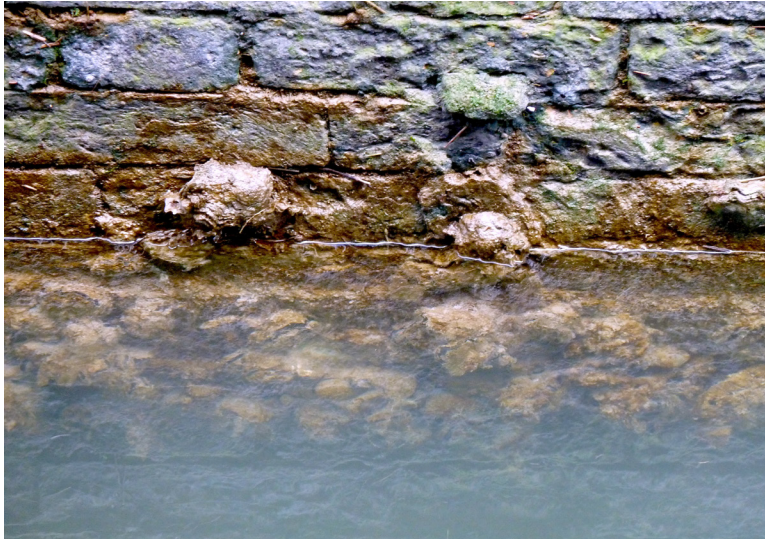
Figure 10.12: Tenuous marine wildlife secure attachment to Venetian brickwork and assimilate its materials to sustain their metabolism. In the process, these organisms transform the building fabric so that it is (re)appropriated into biological structures (as shells), or forms new soils (silt). Photograph, Rachel Armstrong, August 2010.
