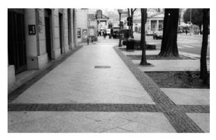
Figure 3. Comacchio (Ferrara), Treponti. The edge of the path was made detectable especially by persons with severe visual problems through paving materials typical in the place of intervention (cobbled – for blind person – and istrian stone – for visually impaired)
