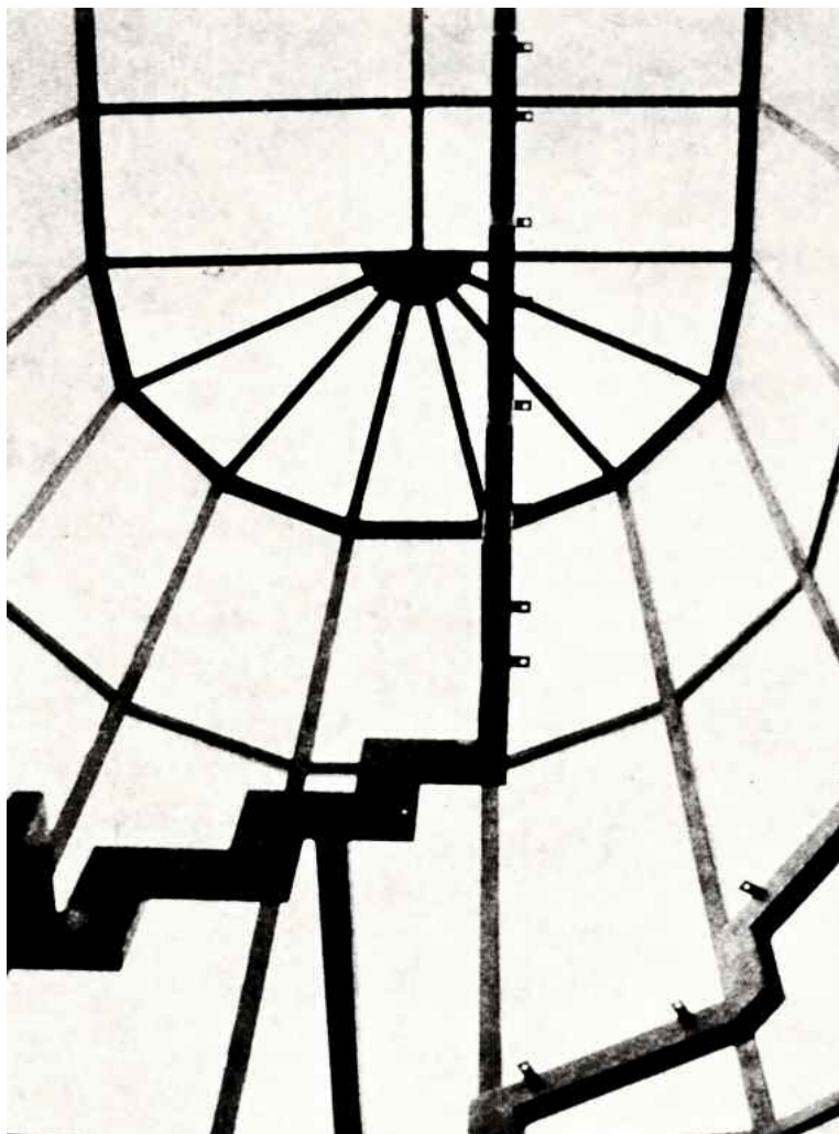
The staircase glazing
