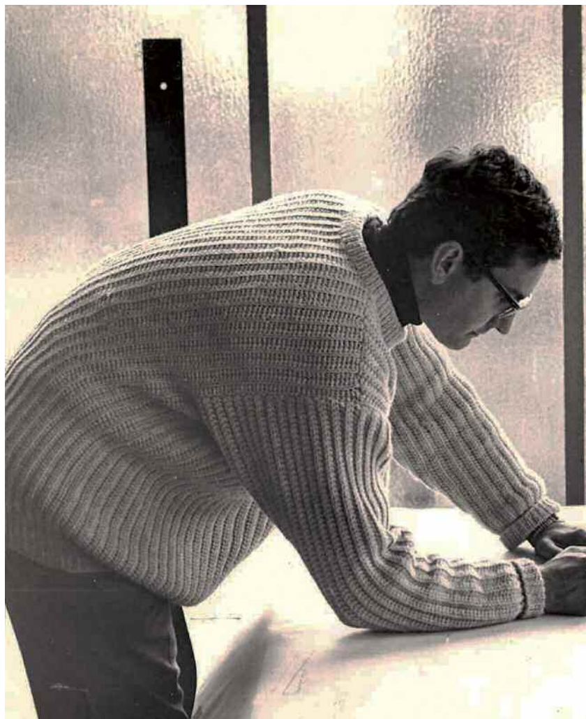
At work on Frei Otto's house and studio, Berlin-Zehlendorf 1967; on the right, a working model
